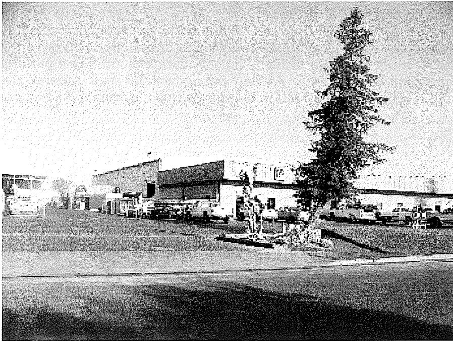
Fruit Growers Supply is a good example of a well designed service commercial use.
